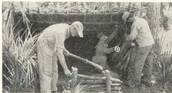
Shelters can be built from whatever jungle growth is at hand. Poles can be lashed together with vines or other plant fibre.
